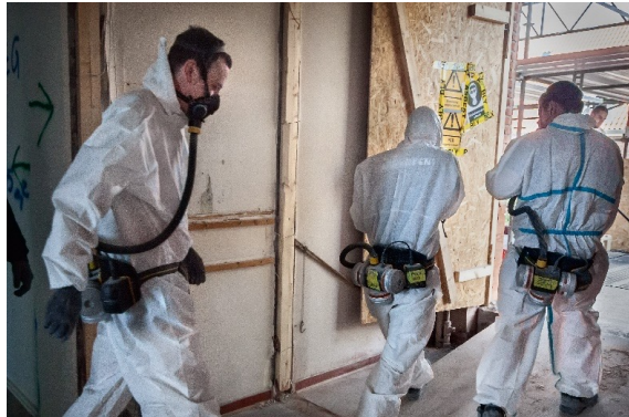
Building decontamination Photo: VCØB
